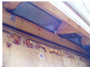
Specimen 4 -The perforated vinyl soffit in conjunction with an insect screen across the threshold of the attic and soffit space
