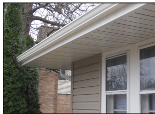
Specimen 1 -Hidden vent soffit
