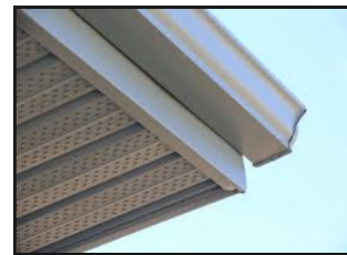
Specimen 3 -Perforated aluminum soffit
