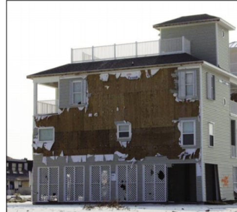
Extensive lost of vinyl siding and housewrap event though high wind panel was used (FEMA 2005)
