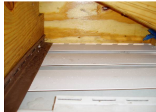
Specimen 5 - deflectors were added to the hidden vent soffits
