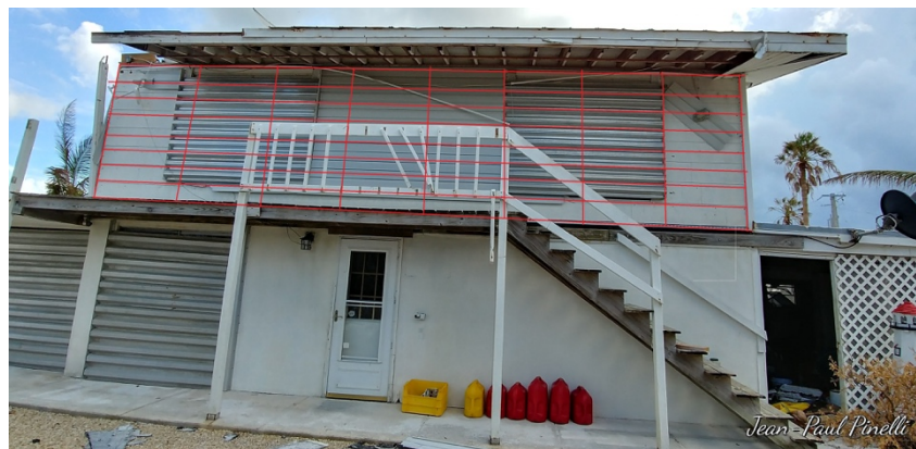
Figure 17. Vinyl siding use and damage levels will be quantified using discrete grids for each wall surface on each story to precisely identify patterns in the locations of failures.
