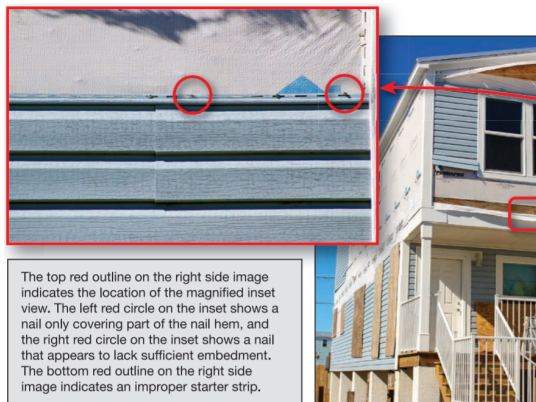
Failure of vinyl siding failure due to nail covering only part of the nail hem, and lack of nail embedment (Fema 2018)
