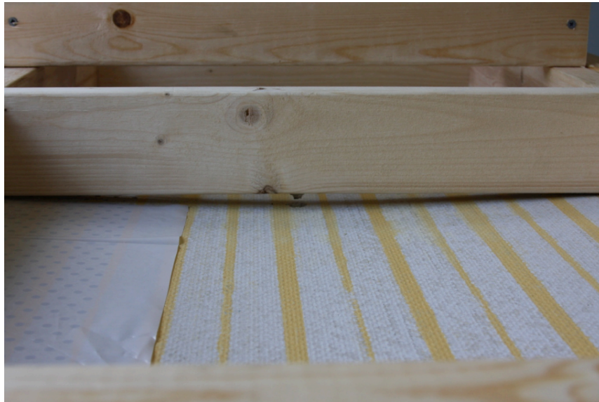
Figure 4. Predominant Failure Mode (Masters and Kiesling 2011)
