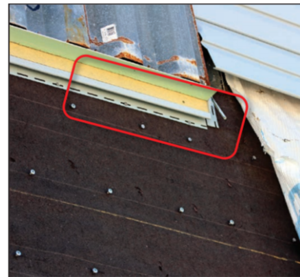
Vinyl siding failure because to lack utility trim under the windows (Fema 2018)
